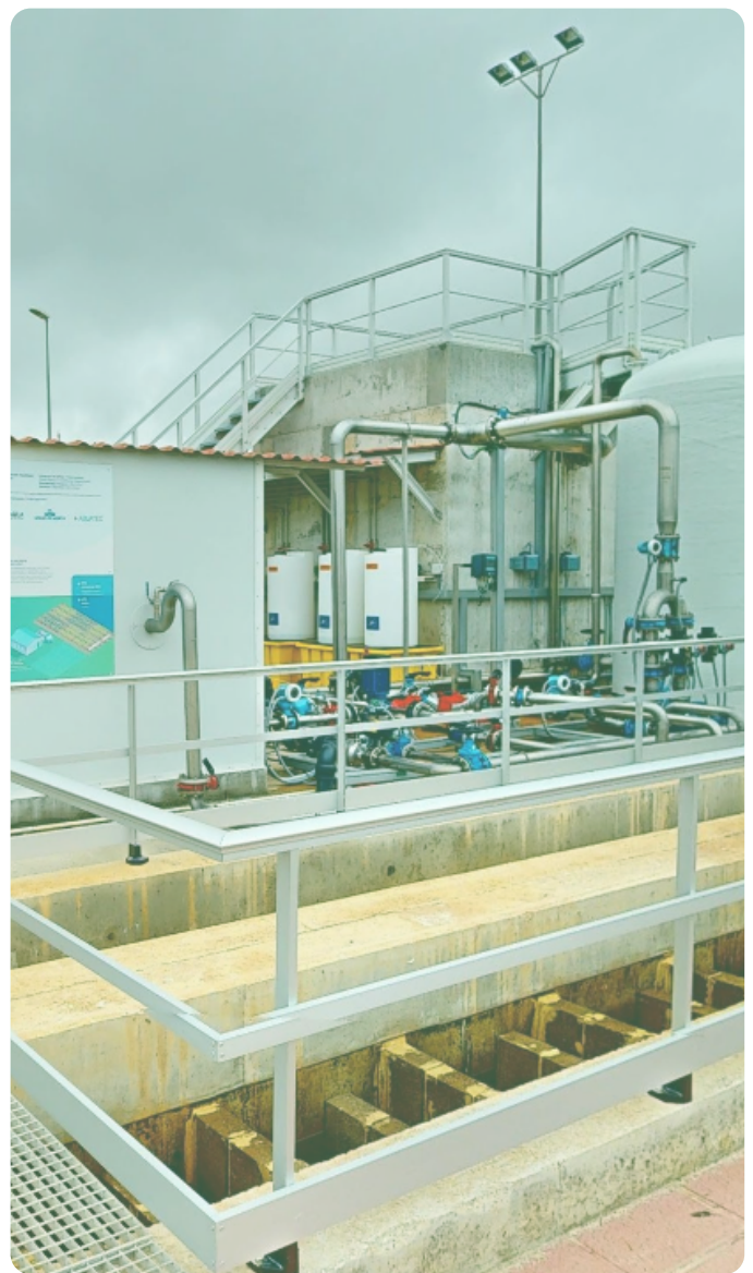
Image 1. LIFE WARRIOR pilot plant. On the left, the shed housing the UV-LED disinfection system and the digital tool, and on the right, the system of reused UF membranes.
