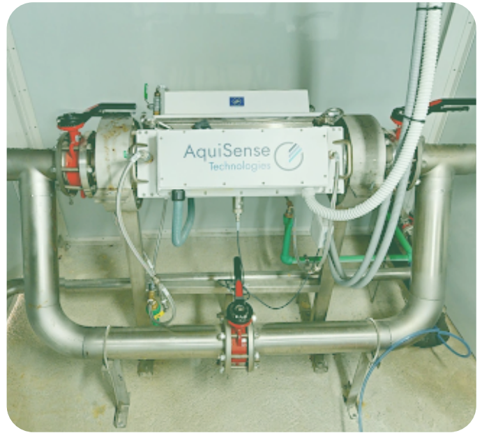
Image 3. UV lamp used in the LIFE WARRIOR pilot plant.
